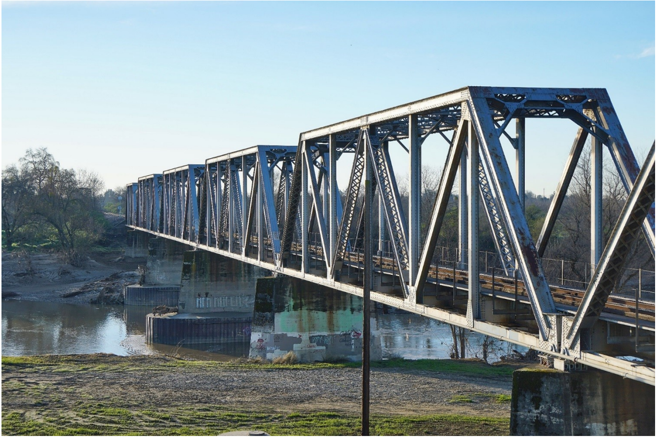
Photo 03: Railroad Bridge in phase 2A
